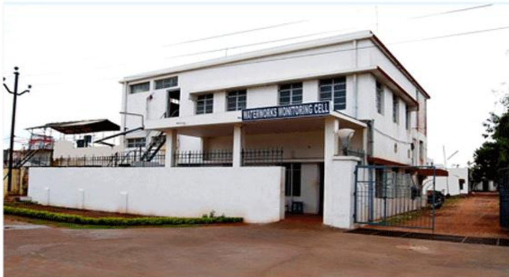
Water Works Monitoring Cell, Palasuni, Bhubaneswar
